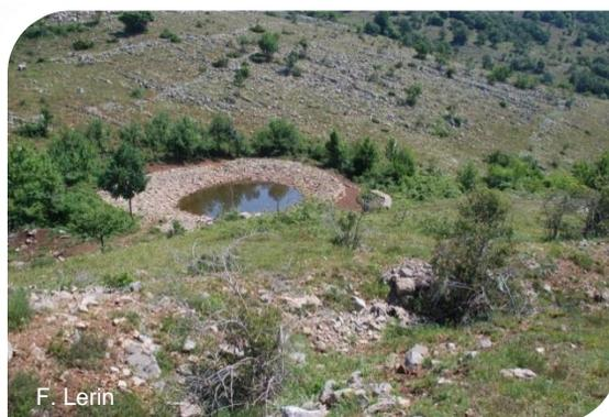
A lavogne was recently built in Cahan. The stock farmers do not use it because it was badly designed and badly built (the plastic waterproofing was made from an unsuitable, fragile material which was quickly torn. A stock farmer explains: *“They issued a call for tender but no one consulted us... they would have been better advised to give us the money and we would have done something useful for our farms.”*
